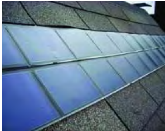
Image 35: Integrated solar panels
